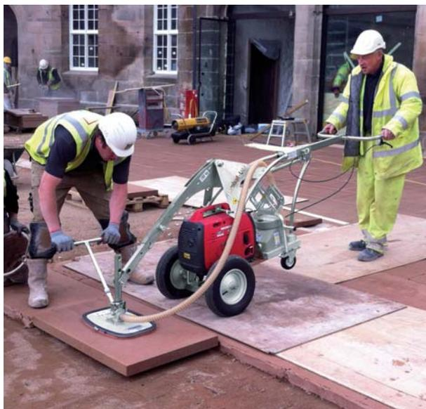
UNIMOBIL UM-VS-S/SE Chariot de pose, Appareil complet
