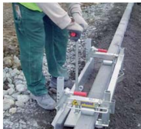
Slipform for Concrete Kerb Backfill GR-150
