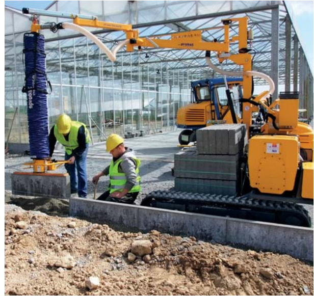
TRANSMOBIL TM Installation Carrier installing kerbs
