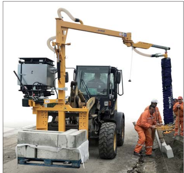
JUMBO-BV-VARIO Vacuum Kerb Stone Installation
