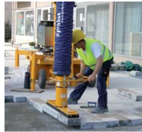
JUMBOMOBIL JM-VARIO Vacuum Slab Laying Machine
