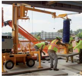
JUMBOMOBIL JM-VARIO Vacuum Slab Laying Machine
