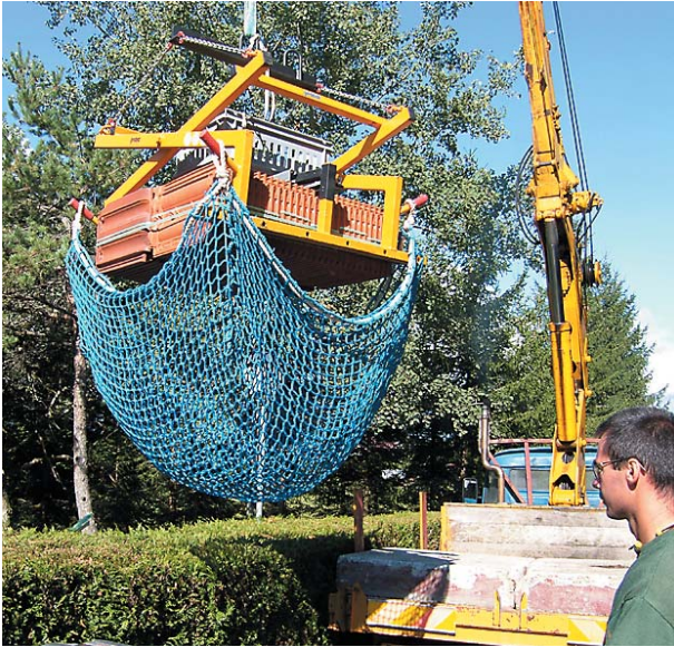
Roofing Element Clamp DEZ-UNI
