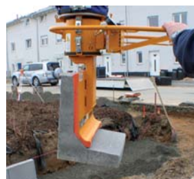
Special suction plate for angular concrete products
