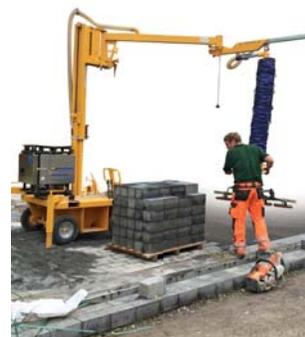
Install concrete slabs, natural stone slabs and large pavers effortlessly and accurately up to 200 kg.
