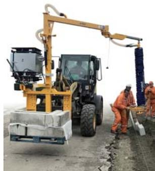
Kerb stone laying directly from the pallet. Lifting & installation all in one operation up to 250 kg.
