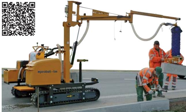
A compact universal machine – transport and handling of palletised building material and vacuum installation all in one. The powerful vacuum laying unit allows the immediate installation of heavy construction elements up to 250 kg – effortless and without physical strain. The chassis with rubber tracks is particularly suitable for uneven terrain.
