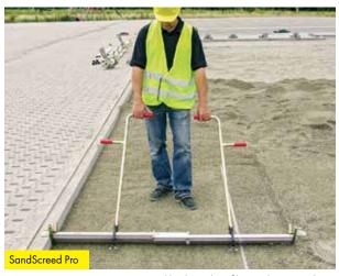
Sickle-shaped profile cuts the material accurately and prevents the TELEPLAN from running upwards.
